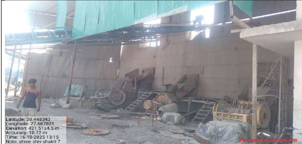
Primary crusher and secondary not covered.
