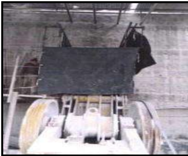
Figure-1: Covering of Primary/Jaw crusher
