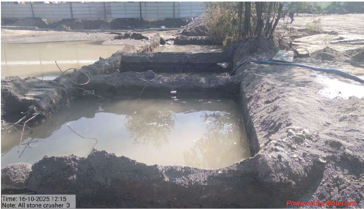
Sedimentation tank
