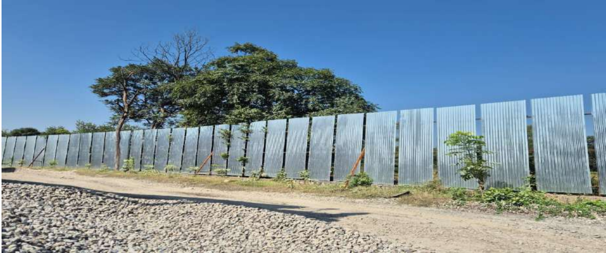
Wind breaking wall.
