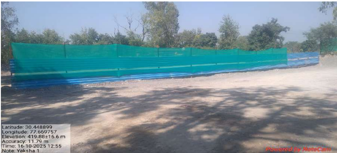
Wind breaking wall
